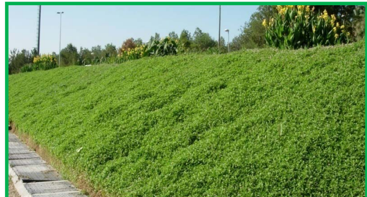
Side of the biological treatment and channel for collecting the treated water
