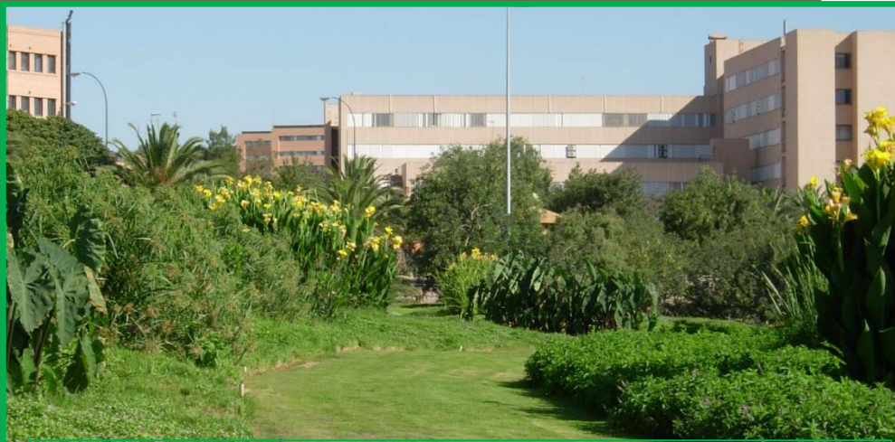
Top view of the biological treatment
